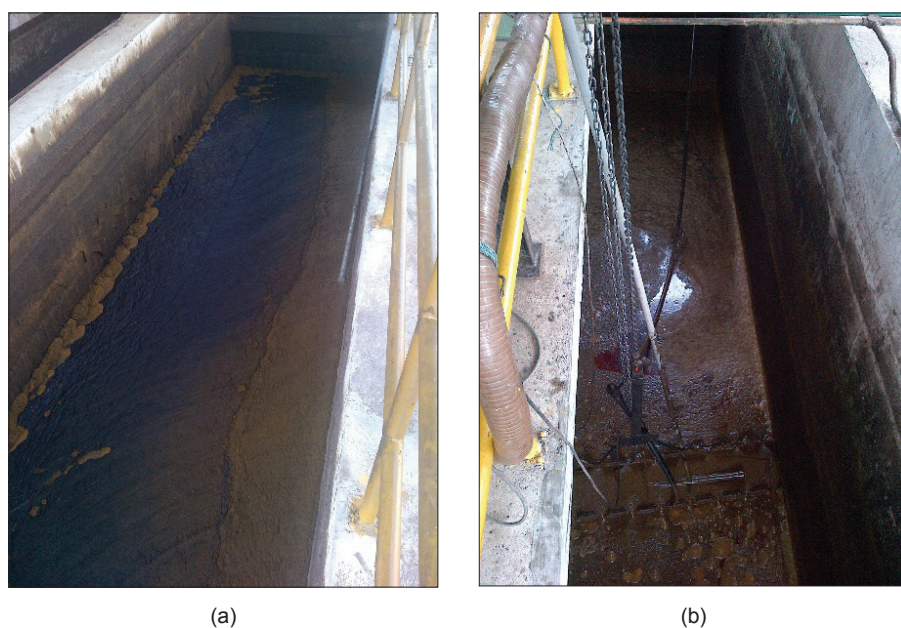
Figure 4. Thick layer of oil formed on the surface of (a) oil separation tank and (b) equalisation tank.
